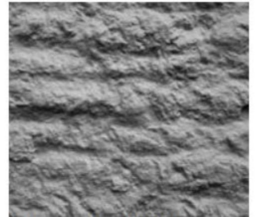
Fig. 6.9: CSP 9 (heavy scarification— rotomilled)
